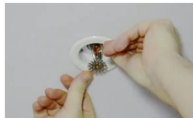
2. Press the escutcheon into place until secured
